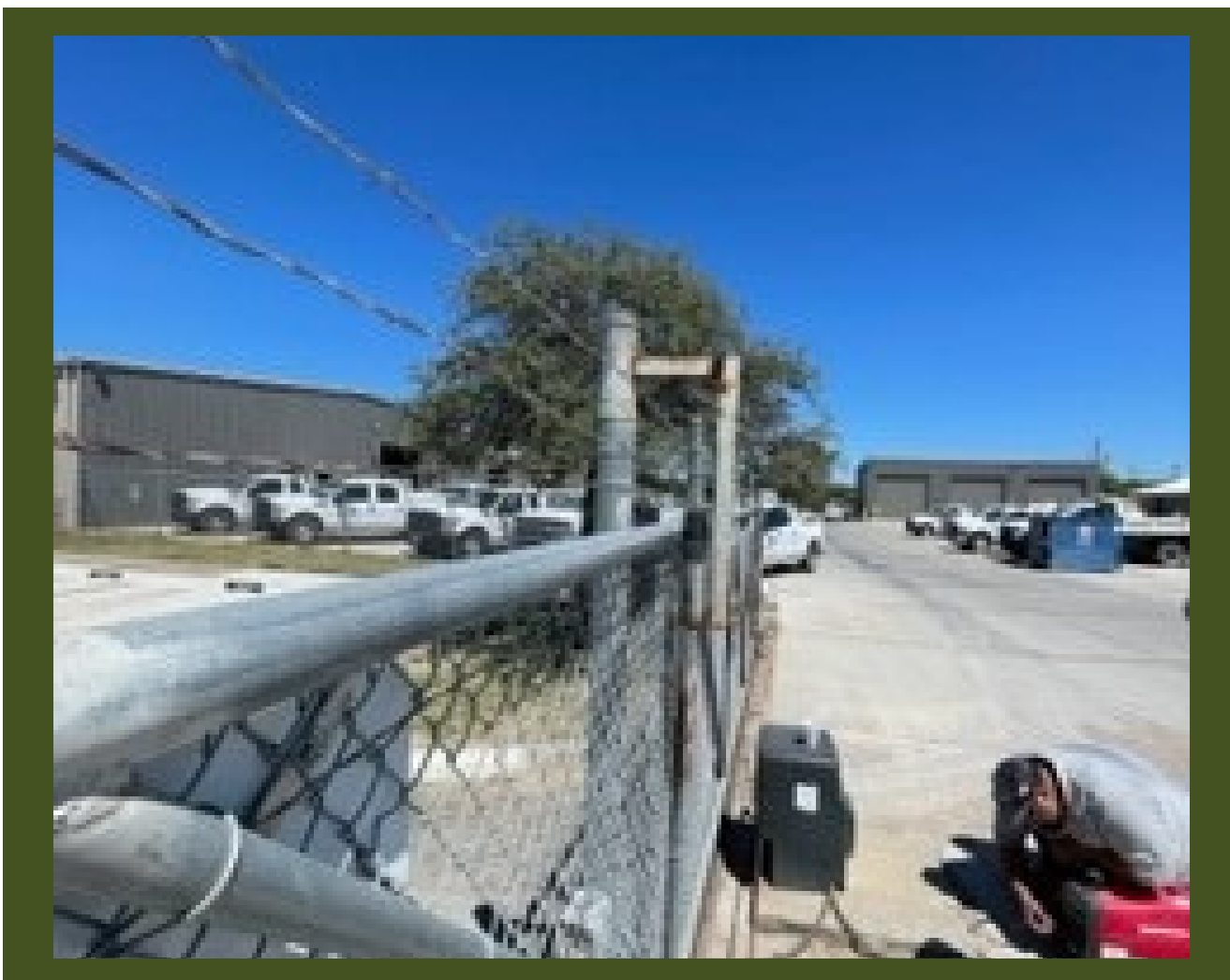
SHOP GATE REPAIR
