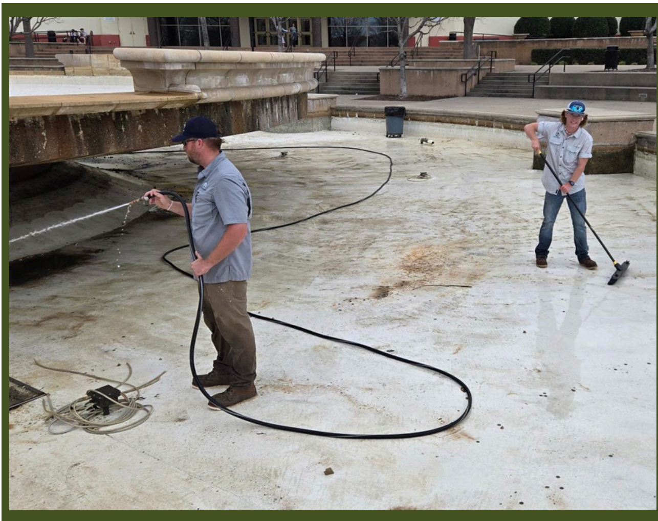
HARBOR FOUNTAIN CLEANING AND LED LIGHTING PROJECT
