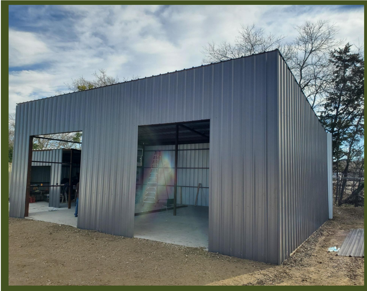
PARK STORAGE BUILDING FABRICATION
