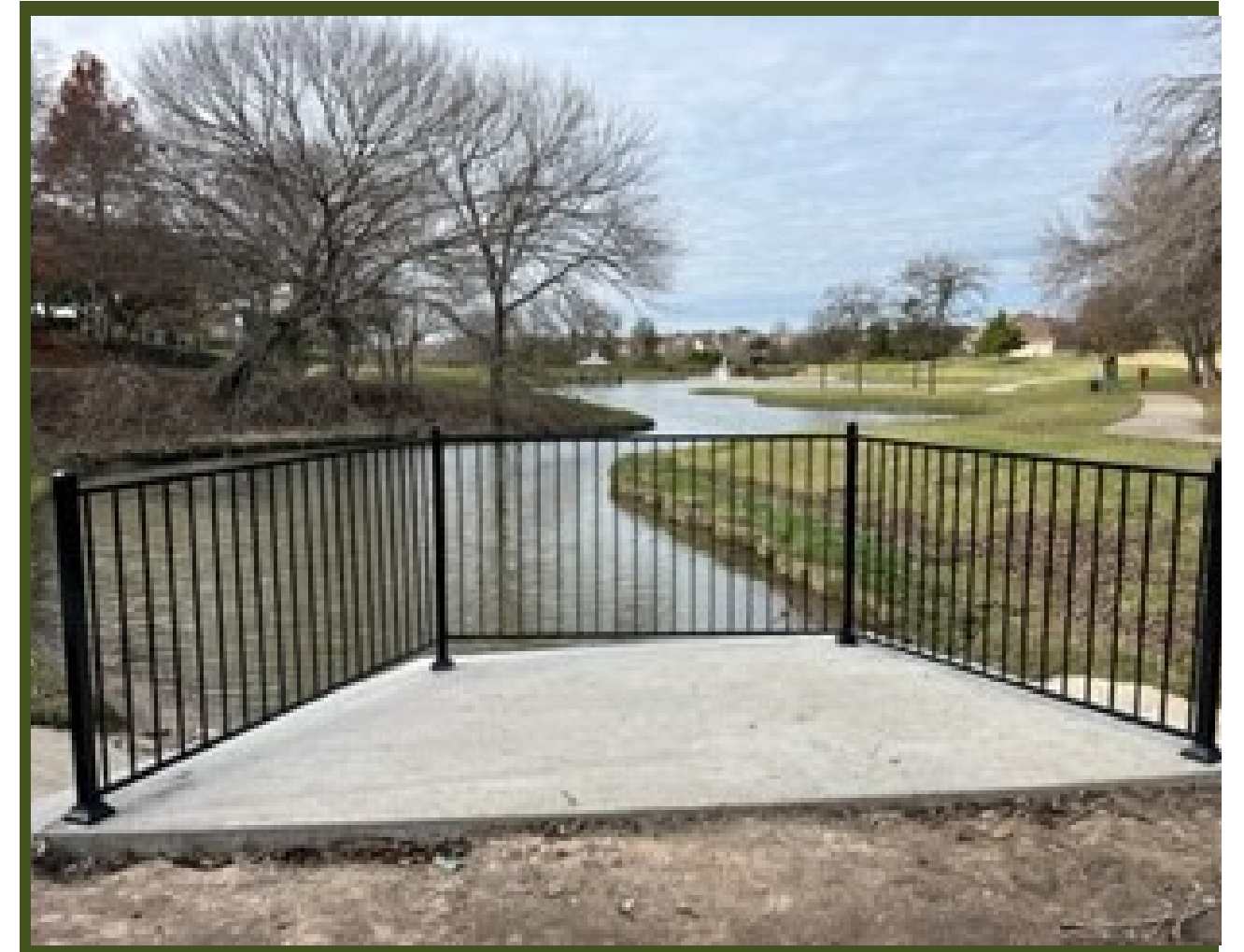
EMERALD BAY METAL FENCE INSTALL
