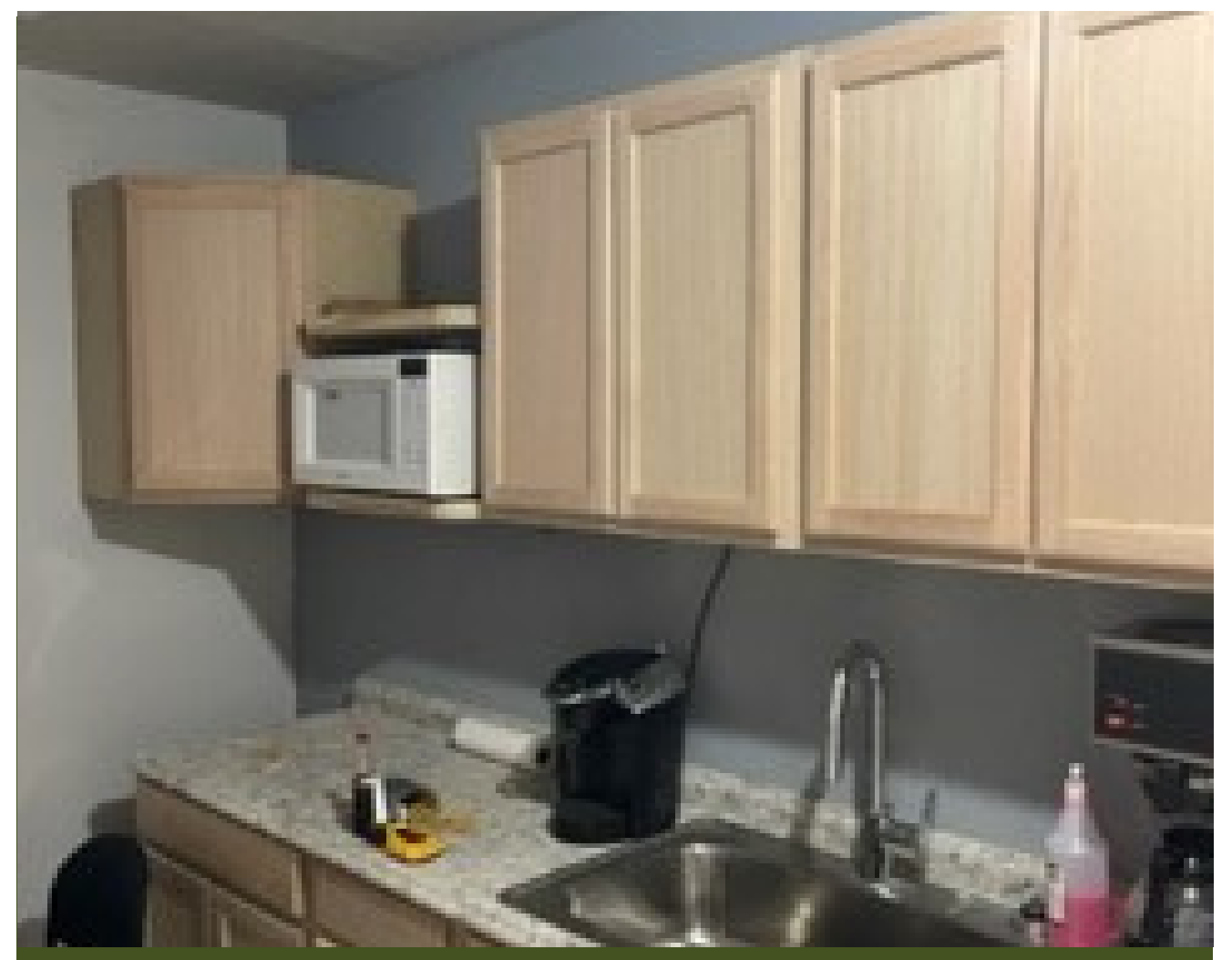
PARKS BUILDING CABINET INSTALL AND PAINTING
