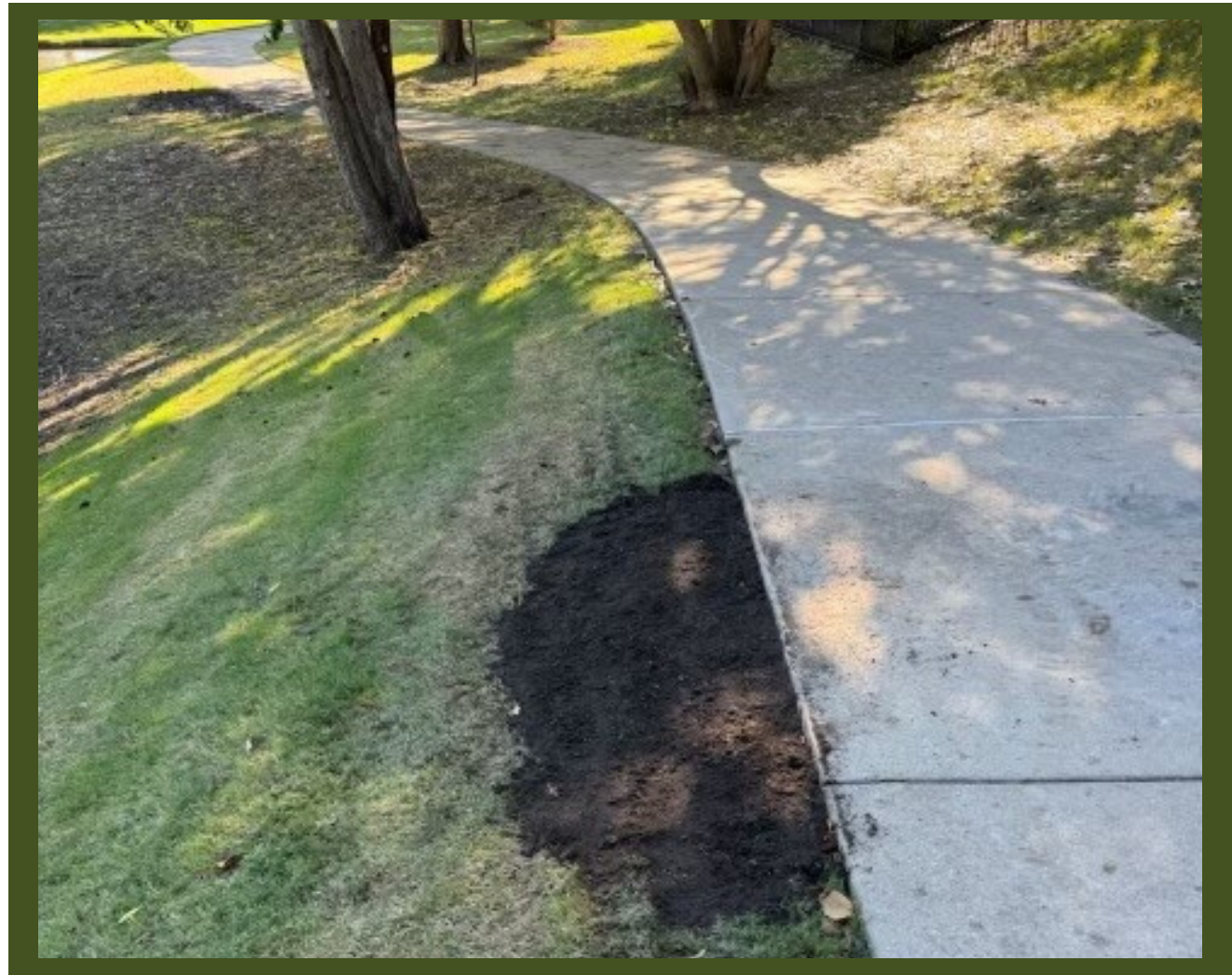
EMERALD BAY SINK HOLE REPAIR AFTER
