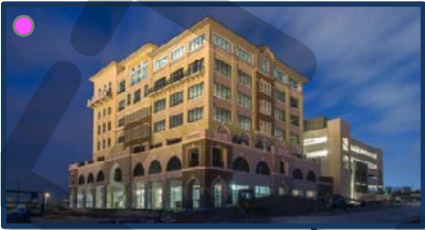
1 Trend Tower Office Building
