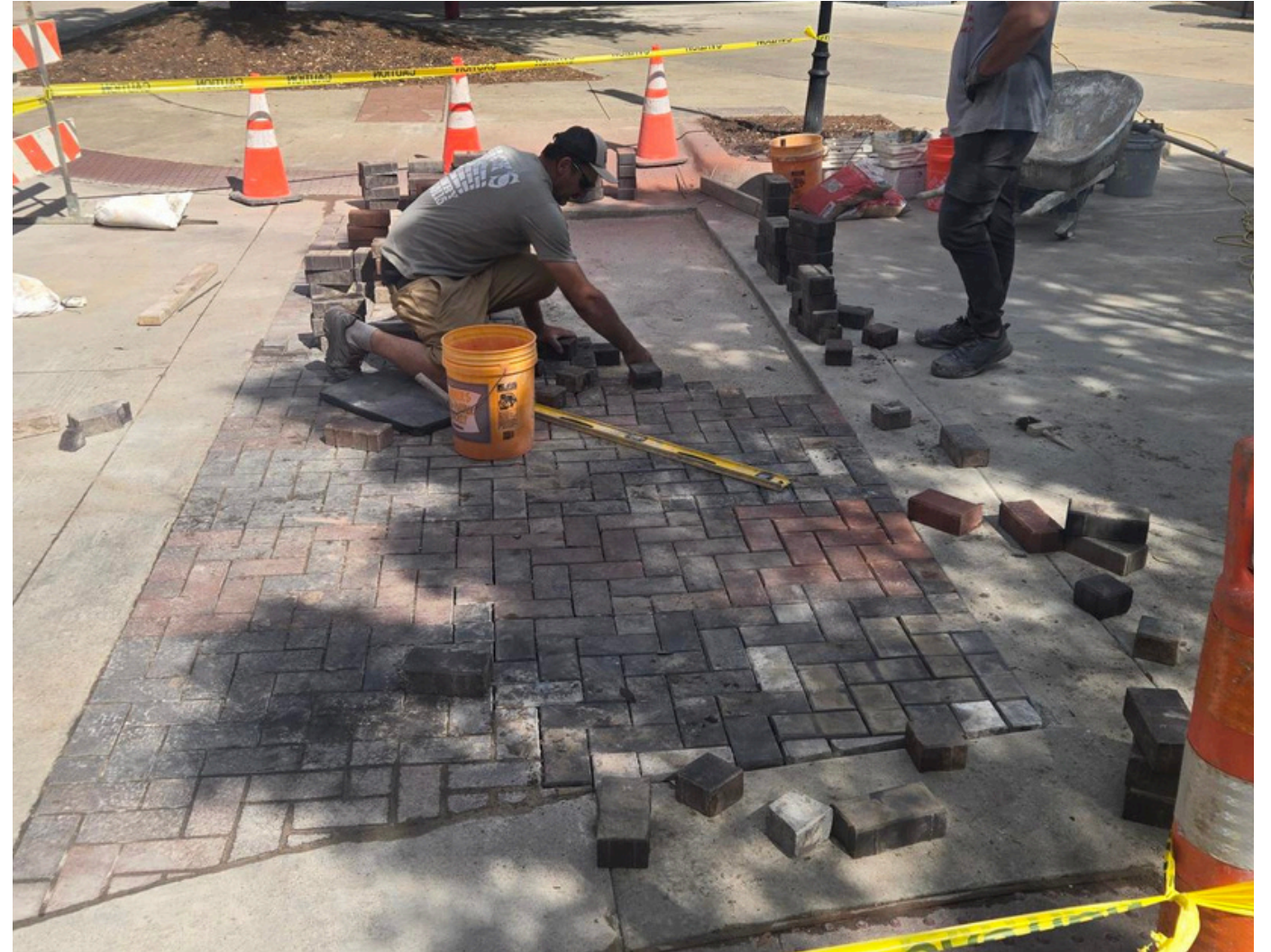
DOWNTOWN CROSSWALK REPAIRS
