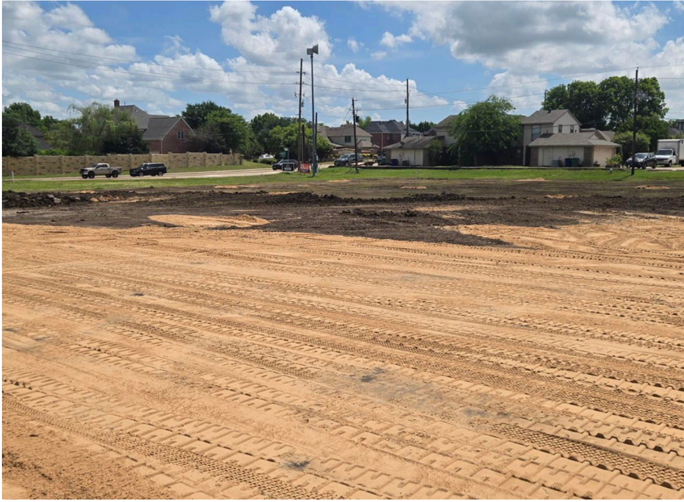
CHANDLERS LANDING FIELD RENOVATION
