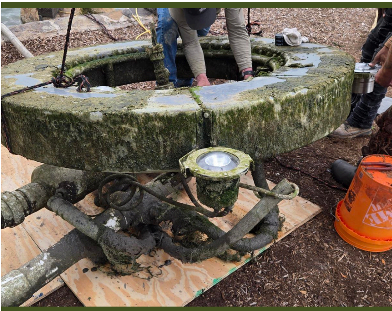
FOUNTAIN LIGHT REPAIRS
