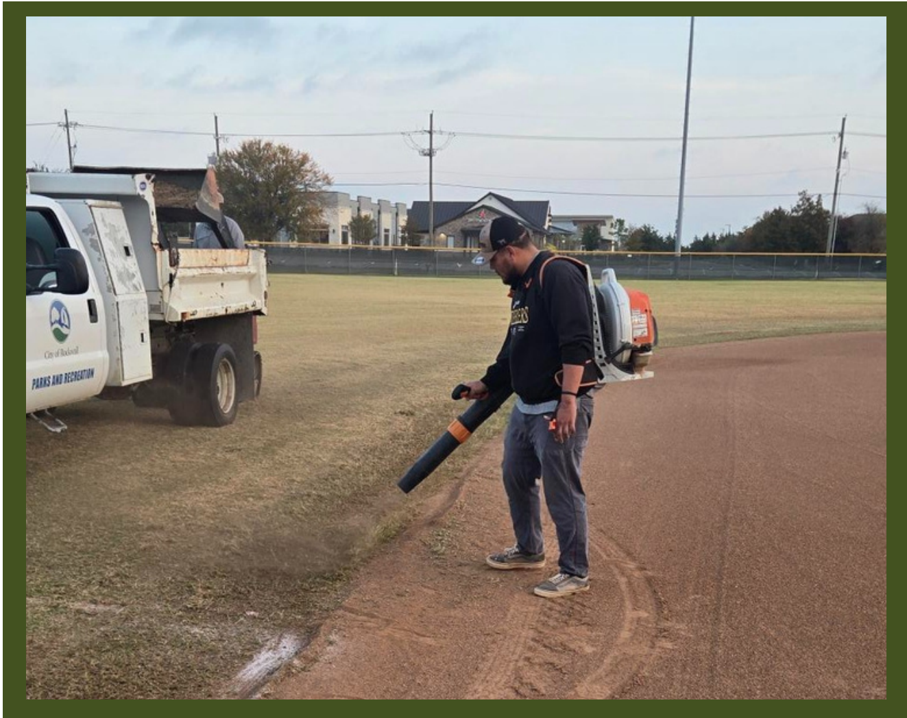
LEON TUTTLE FIELD RENOVATIONS
