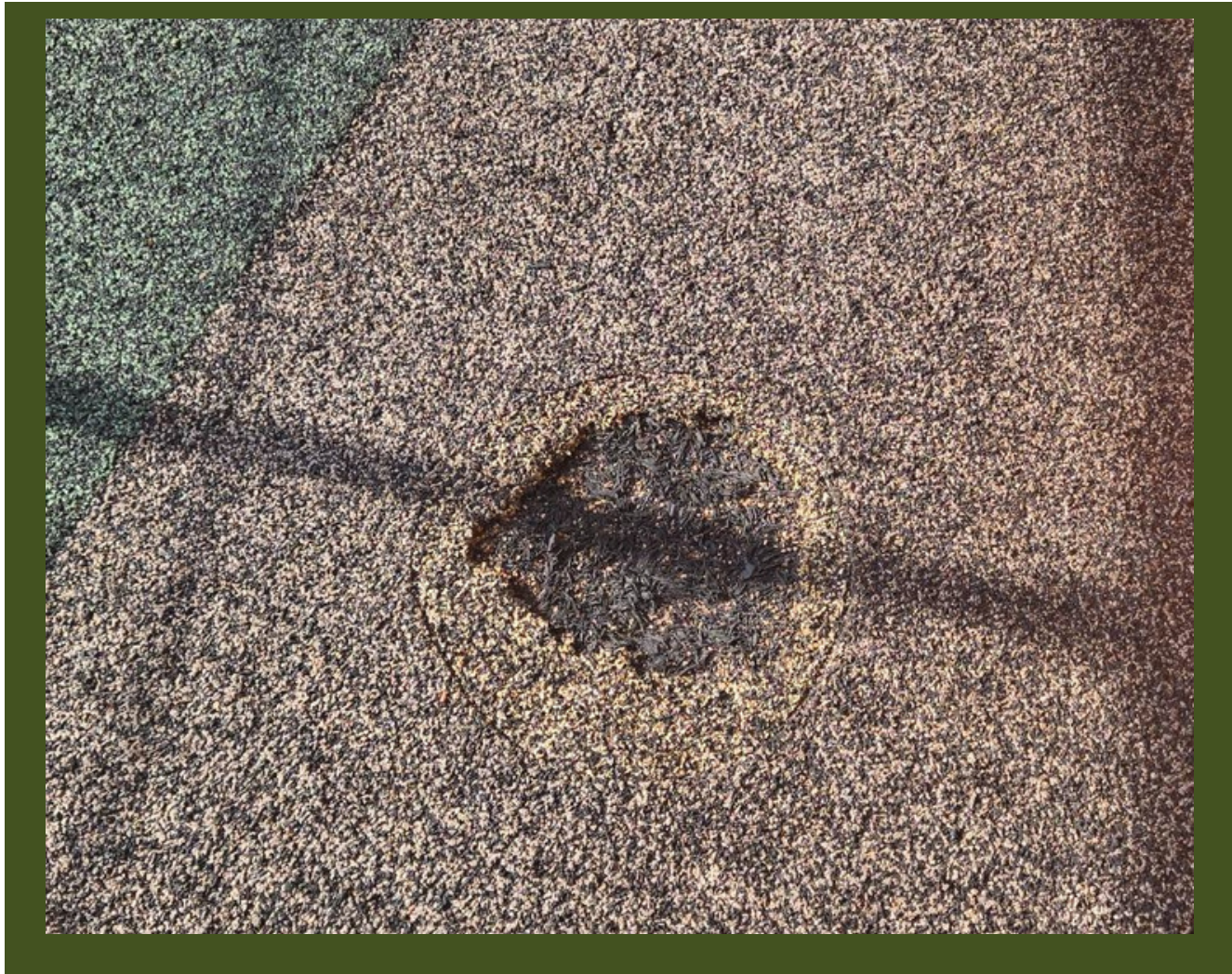
YELLOWJACKET PLAYGROUND SURFACE REPAIRS
