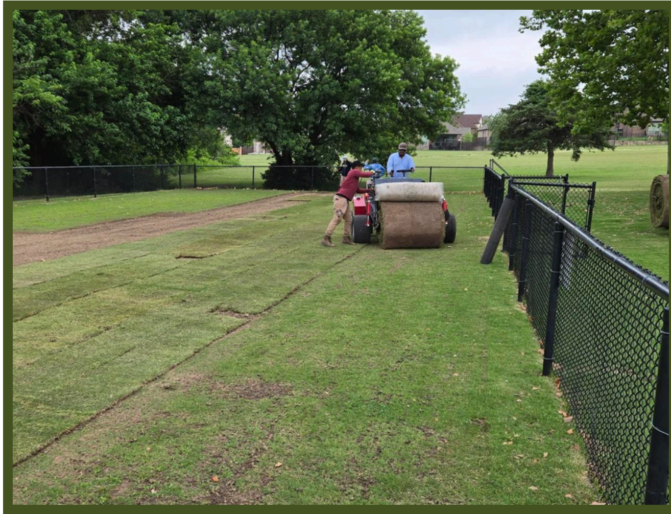
NORTHSHORE SOCCER REFURB
