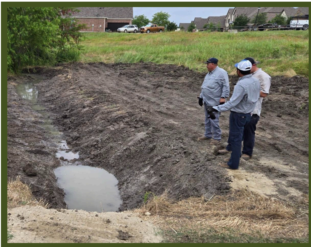
BREEZY HILL DRAINAGE WORK
