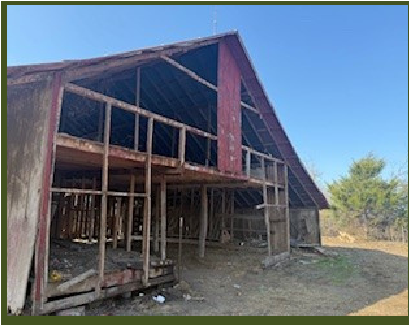
FM 1141 / ALMA WILLIAMS PARK BARN REMOVAL
