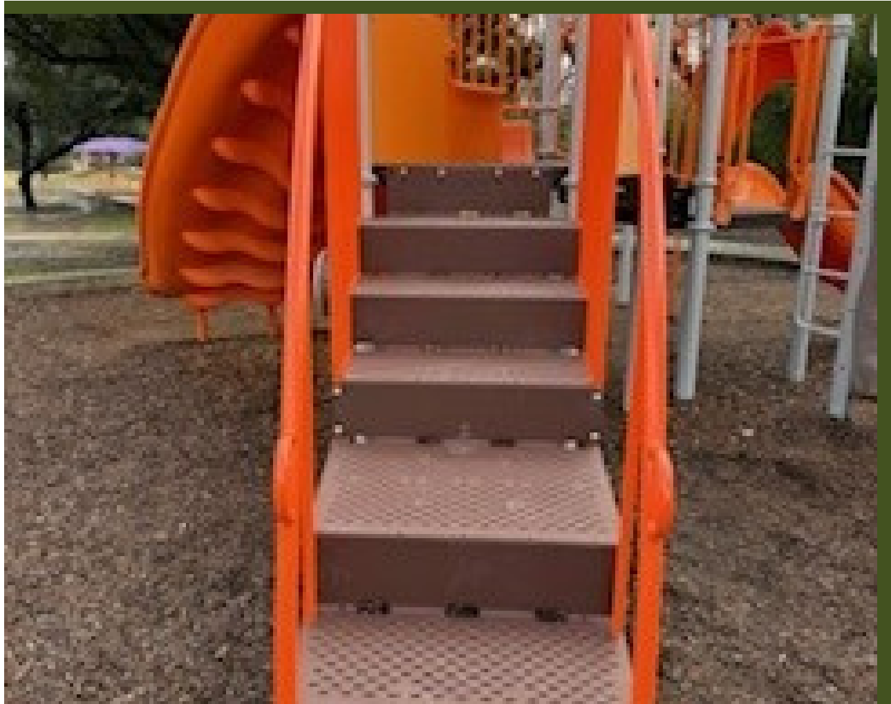
LOFLAND PLAYGROUND STAIR REPLACEMENT
