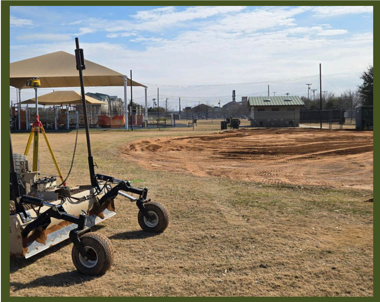
YELLOWJACKET FIELD RENOVATIONS
