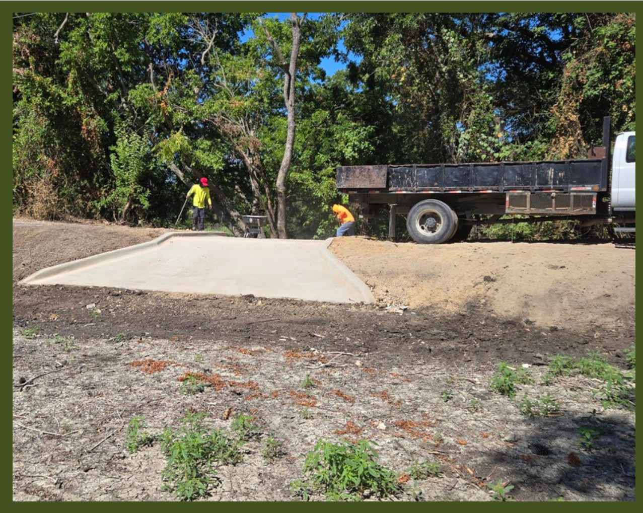
JEWEL PARK DAM AND SPILLWAY REPAIR
