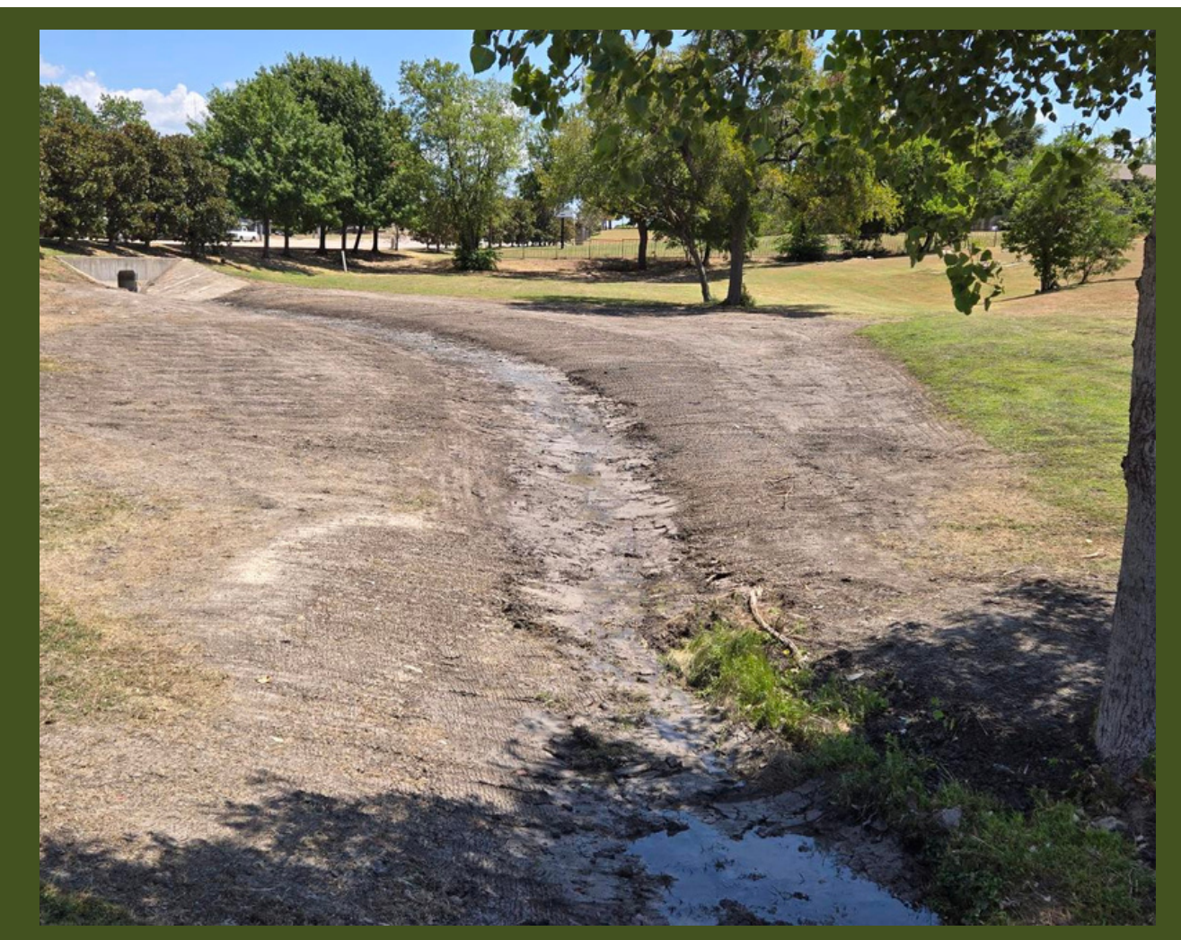
205 CEMETERY DRAINAGE REPAIRS
