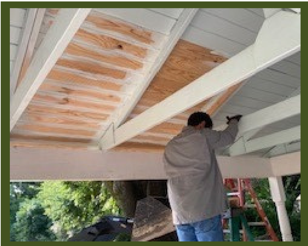
LOFLAND PAVILION REPAIRS
