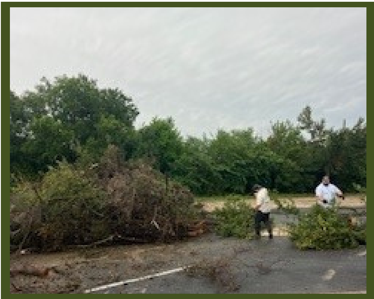
MYERS STORM DAMAGE CLEAN UP
