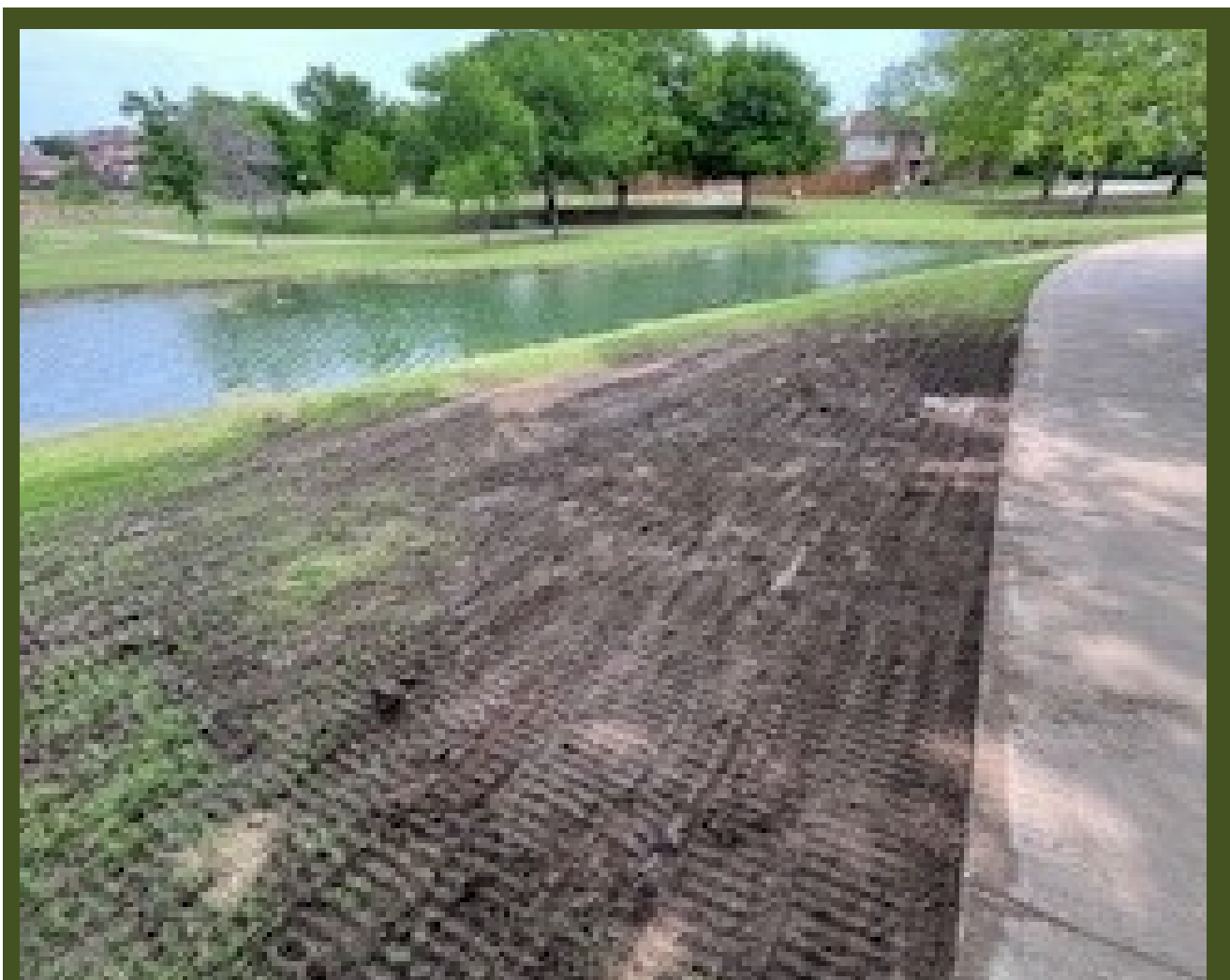
EMERALD BAY EROSION REPAIR
